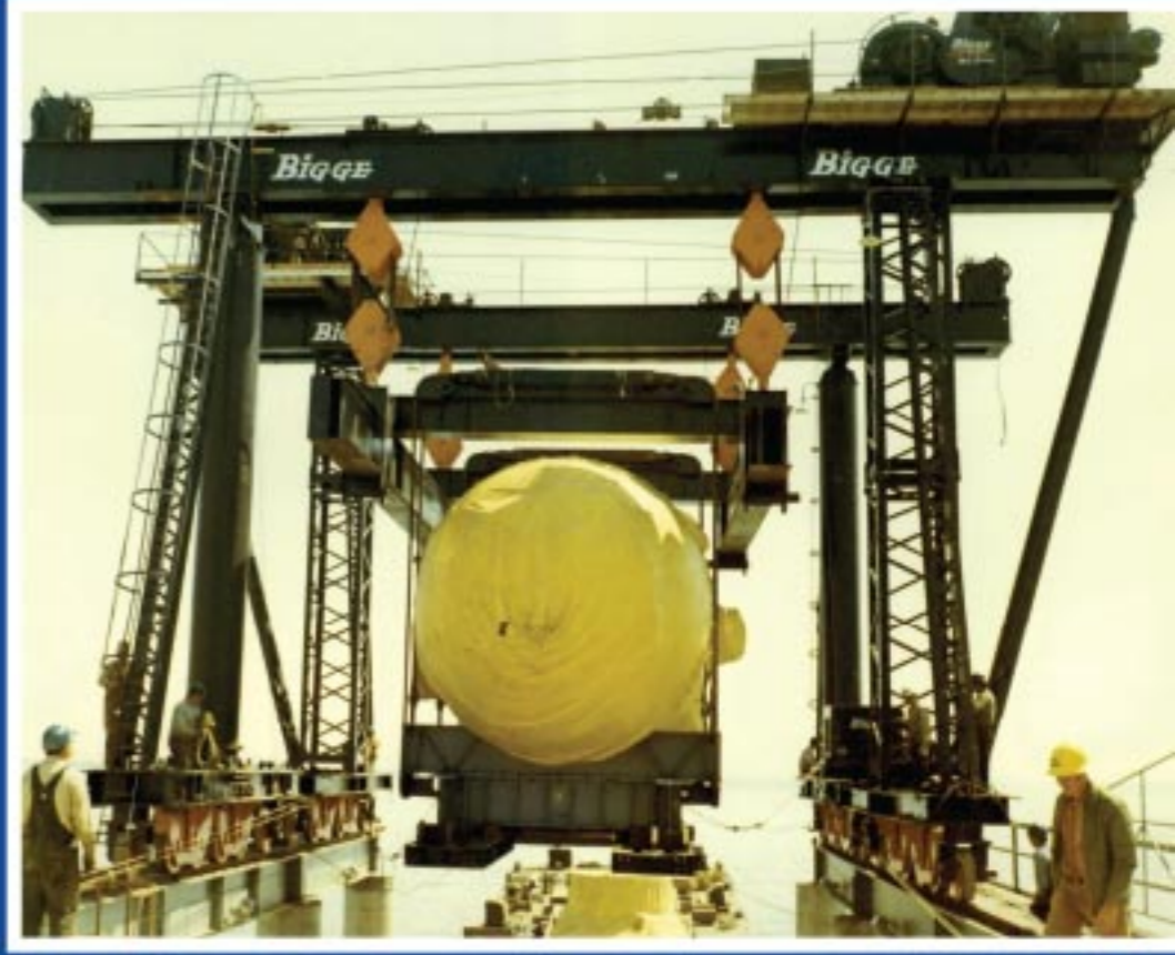
Diablo Canyon Reactor Moving Reactor Vessel Head into Containment
