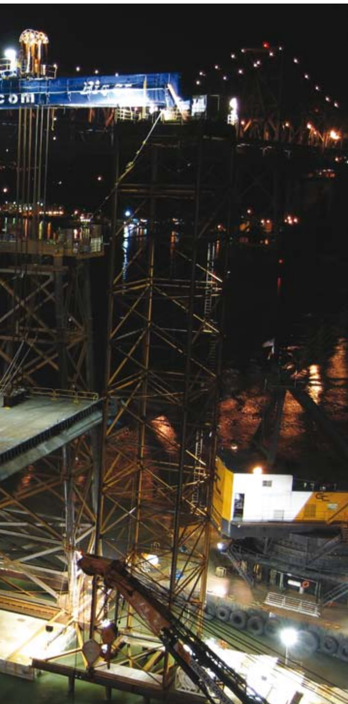
Bigge uses a strand jacking systems to lift a 2,000 ton section on the new San Francisco/Oakland Bay Bridge.
