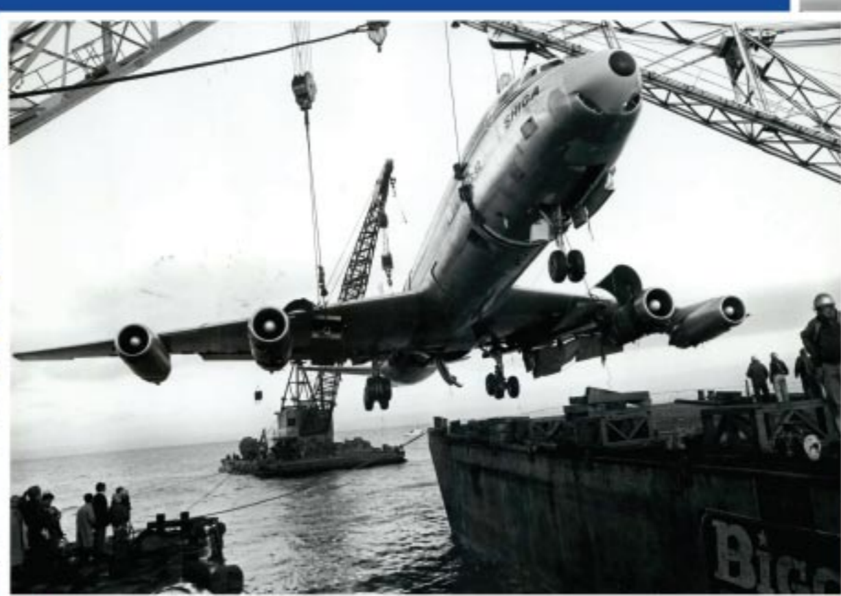
Caption No. 3 (Photo 11416F-20) The third lift point was immediately forward of the tail assembly. Bigge riggers adjust where ailing and through impossible wet the base of the San Mateo bridge shows, which Shiga barely cleared by the narrowest.
