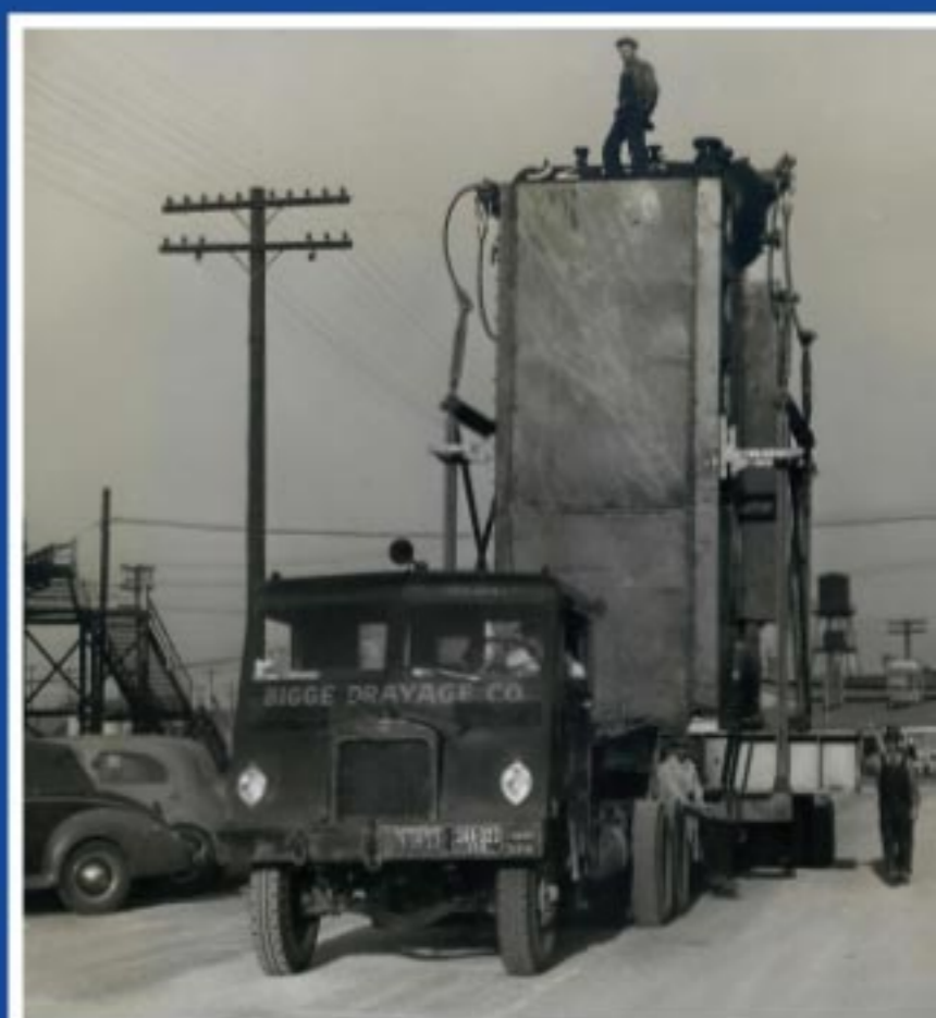
Moore Dry Dock Hauling boiler for Victory Ship, West Oakland Yard
