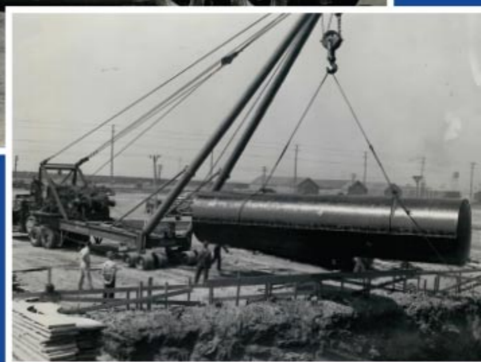
Placing Tanks for Key System Oakland, CA
