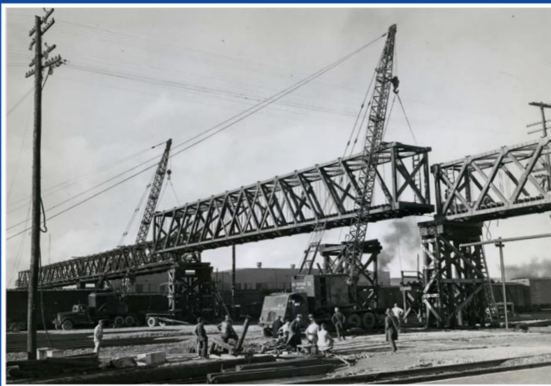
Tressel Assembly Richmond Ship Yard
