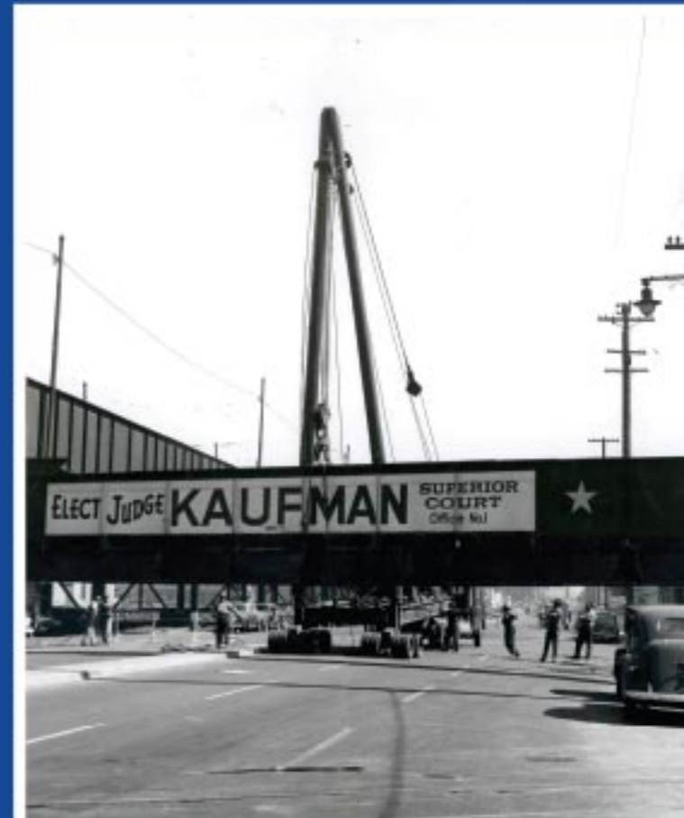
Overpass Removal 3rd Street - San Francisco, CA
