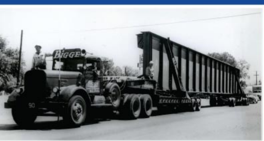
Feather River Bridge 10'9" x 97'6" x 41-ton girder hauling
