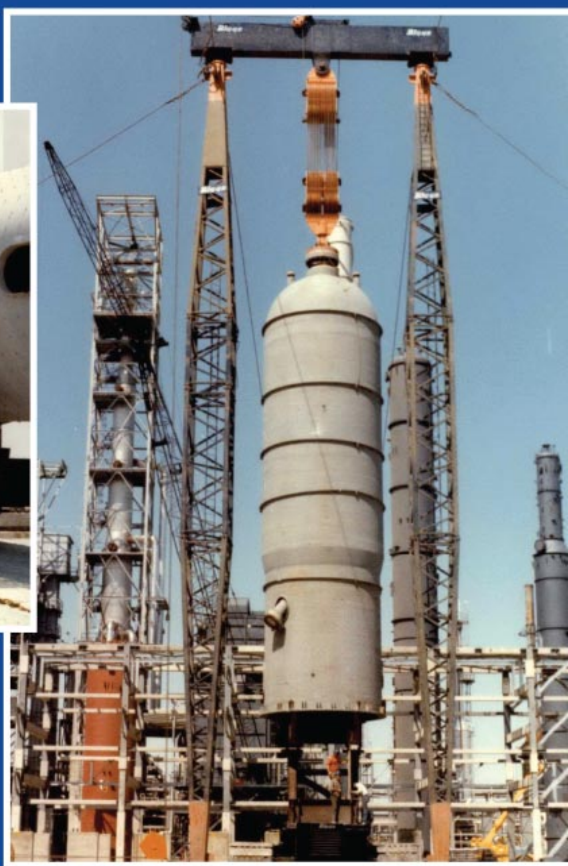
Tosco Avon Refinery 200-ton tower lift
