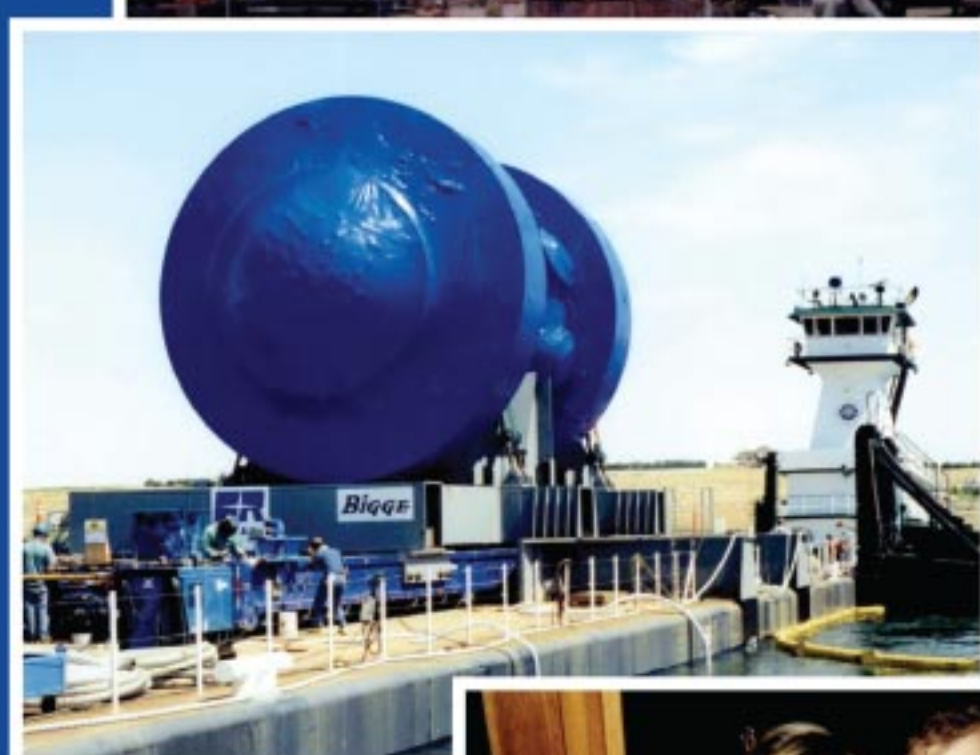
SMUD Nuclear reactor hauling – Rancho Seco
