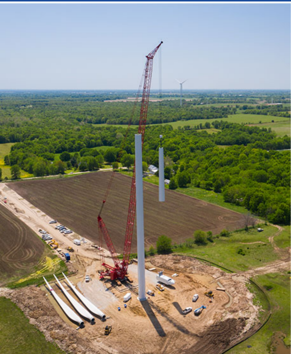
Wind Turbine Construction Missouri
