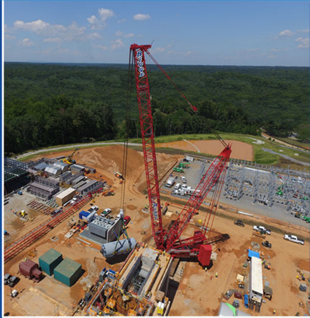
Generator Hoist South Carolina
